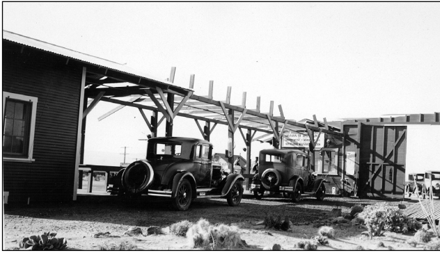
Damage at the quarantine station at Yermo after a wind storm, January 10, 1933. SBd 31-H, California Highway Department.
