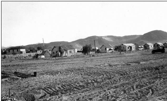
Figure 20. Ludlow highway maintenance yard, ca. 1930. SBd 58-H. California Highway Department.
