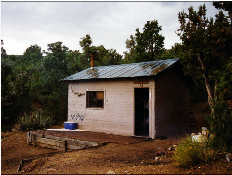
Jim Winkler cabin, Mid Hills, 1994. R.E. Reynolds photo.
