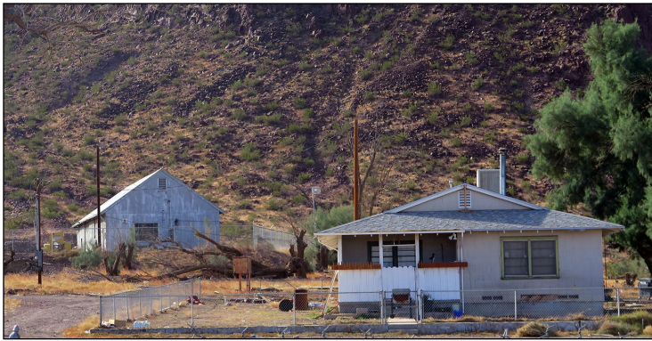
Figure 12. Home and barn in Newberry Springs, 2023. D.M. Miller photo.
