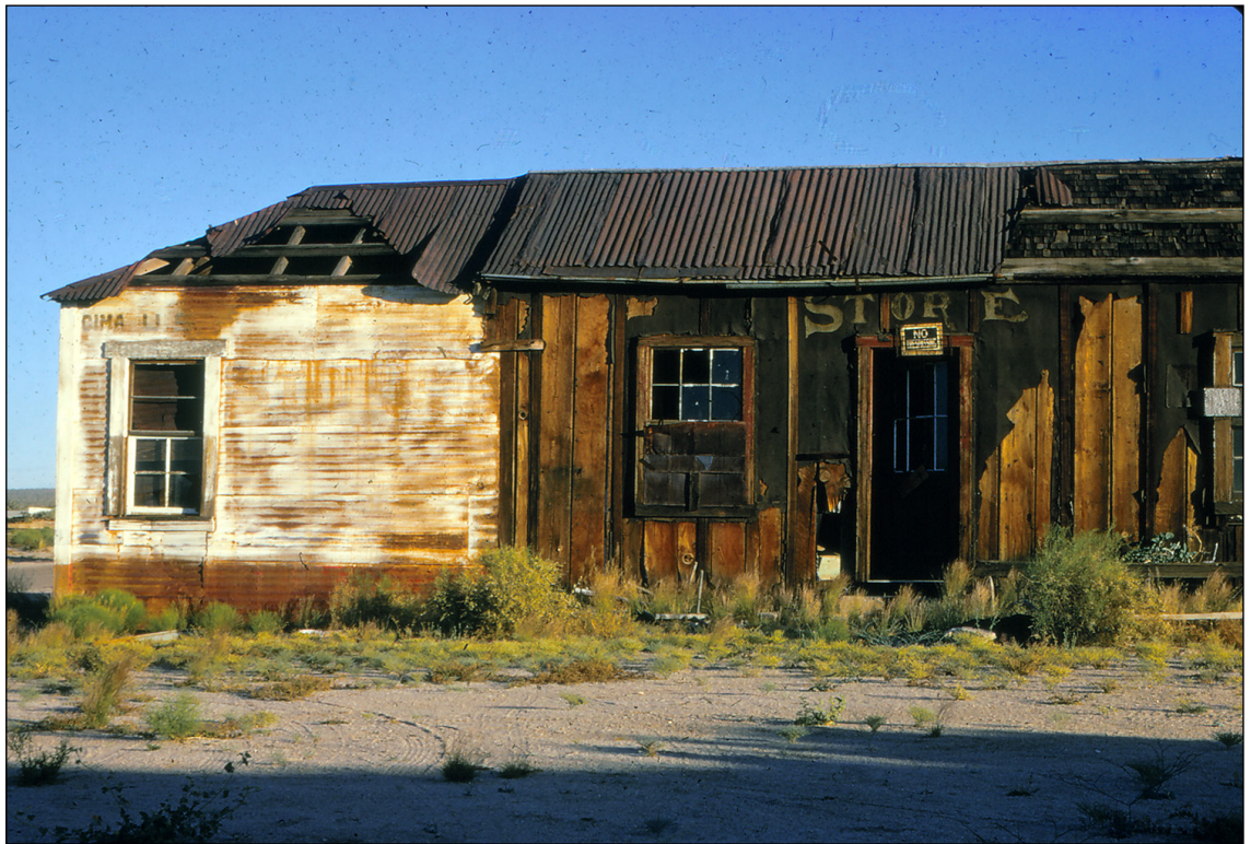
Cima Store (established 1900) and post office (established 1905). R.E. Reynolds photos, 1973.
