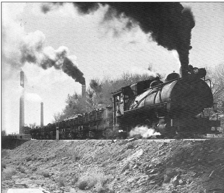
Figure 18. Mojave and Northern backing into Leon Plant. Myrick (1963:865); Southwestern Portland Cement Company collection.
