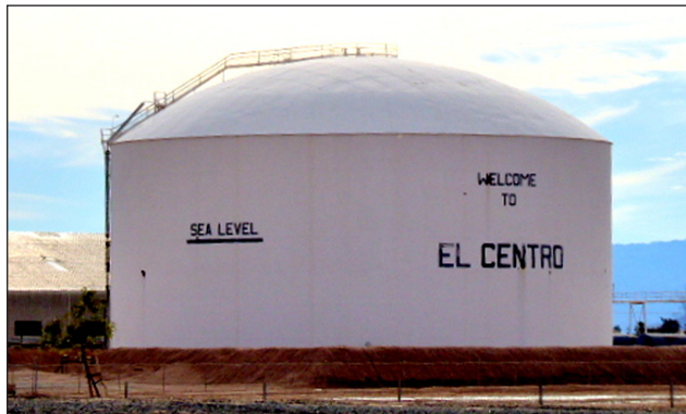
Figure 17. Water Tank at El Centro. © W. J. Elliott, 1-28-2024.
